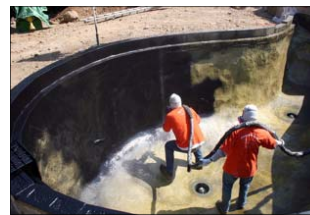
August 5 - First coat of polyurea is sprayed on.
