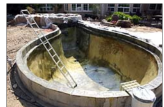
August 4 - Epoxy primer soaks into the concrete and hardens.
