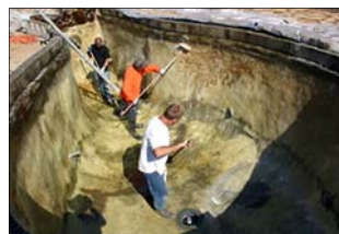
August 4 - Workers apply the epoxy primer.
