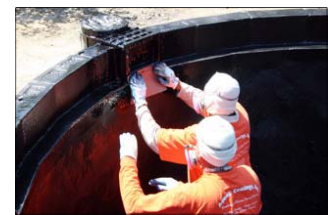
August 5 - Geotextile material is applied around skimmer.
