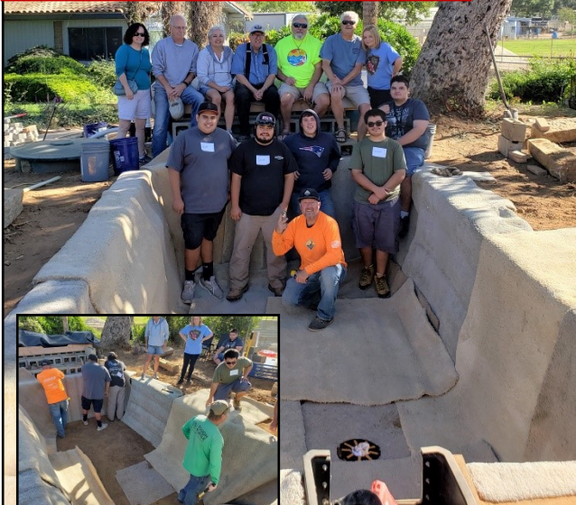
A Group Of Workers Finished the Carpet Layer.
