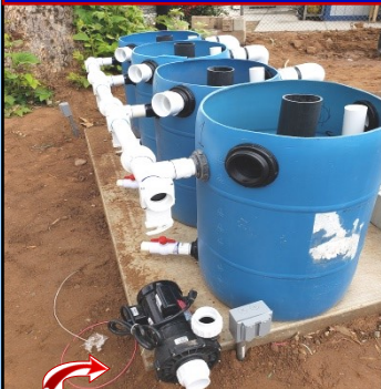
1/4 hp Pump Pushes 5,300 Gallons of Water Per-Hour.
