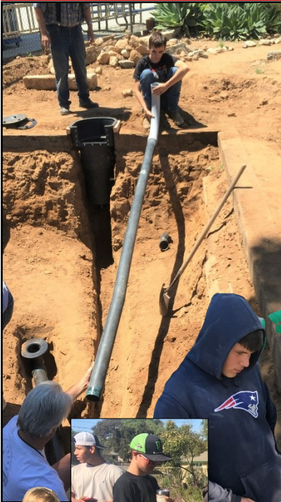
Co-ordinating plumbing between Jack S. and Rob, IKS.
