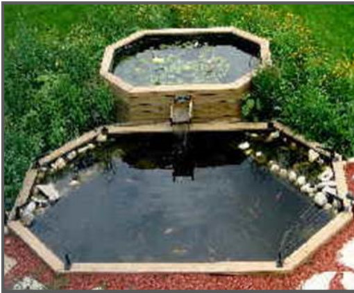
Figure 2: Entire filter system hidden in plain sight. The top pond is actually the anoxic
